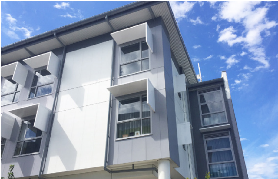
INEX>RENDERBOARD fitted smooth side out with 'V' joints and paint finish.
