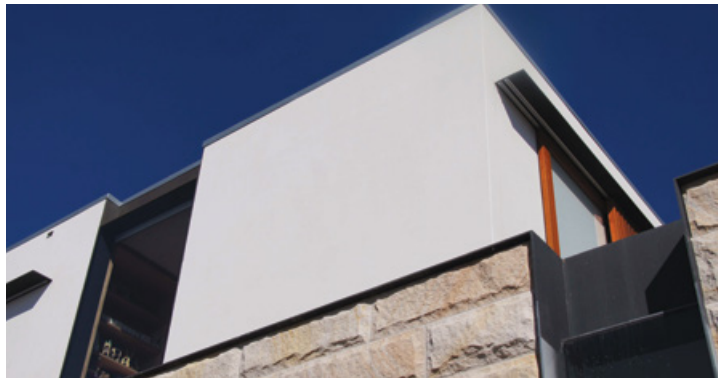
INEX>RENDERBOARD fitted smooth side out with 'V' joints and a clear finish.
