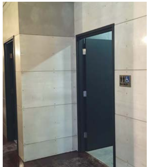
INEX>WALLBOARD 12 with arris edged butt joints and clear seal.
